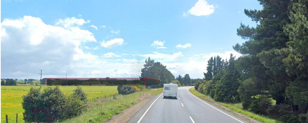
Figure 3 – View from SH6 toward the Terminal Substation
